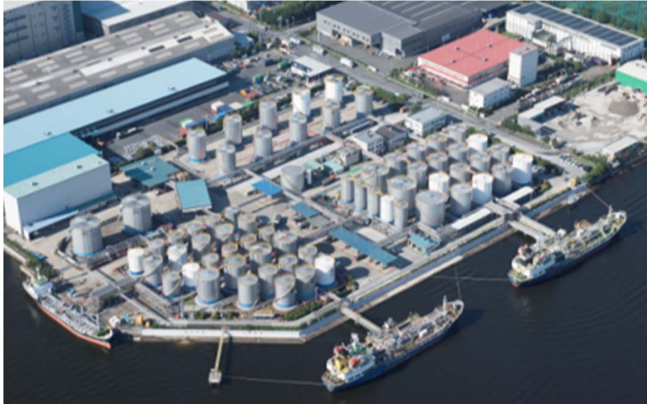
Terminal has 65 bonded storage tanks with various volumes, capable of holding chemicals with different grades and properties
