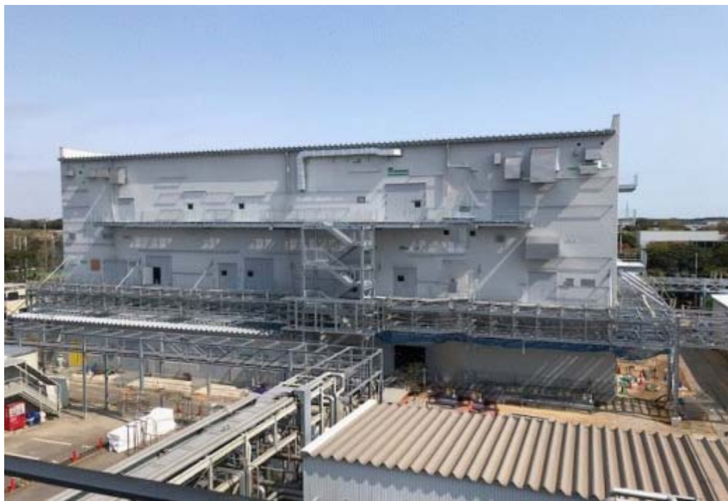
【Construction status】 as of 2021 Apr 17
