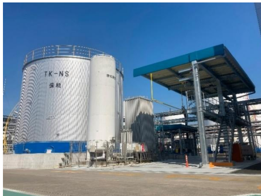
Takahama Tank Terminal Start of Operation of the Dedicated Inorganic Chemical Tank (Completed in June 2025)
